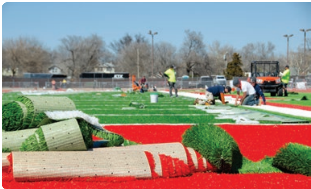
▲ Hoyt Athletic Field turf in Adair-Austin Stadium got a makeover with a brand-new synthetic KTX Blitz 48 turf system with a combination of slit film and high micron monofilament fibers in one system from Kansas Turf, LLC.
